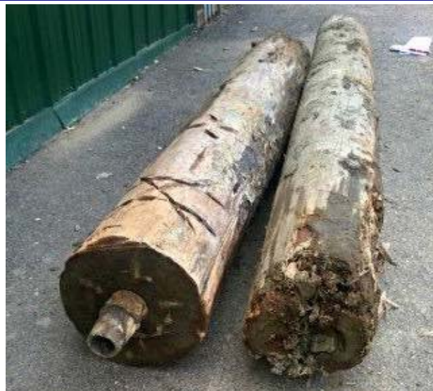
Long-inactive Civil War era wooden pipe discovered during new pipe installation on Hammond Street
